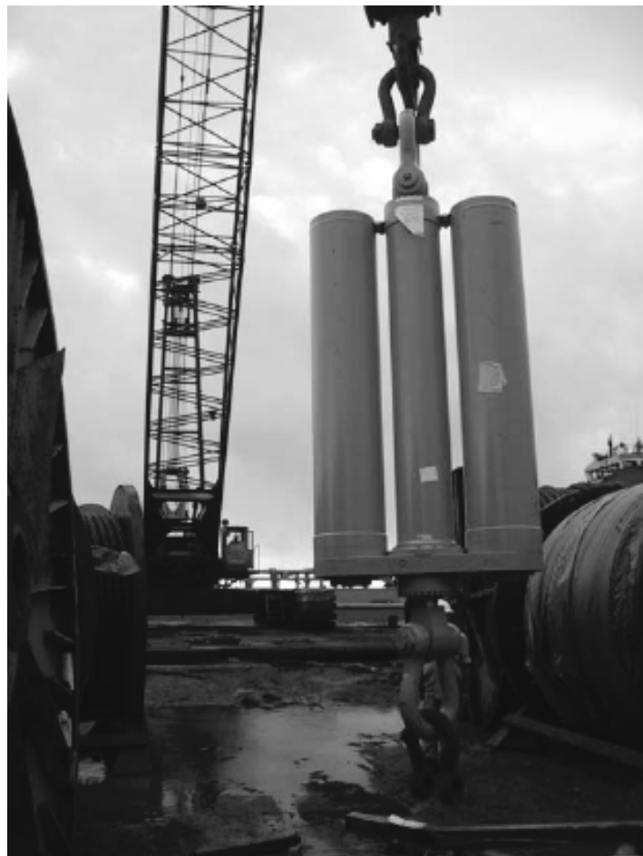
Fig. 7. An example of Passive Heave Compensation use during lifting operations [14]
