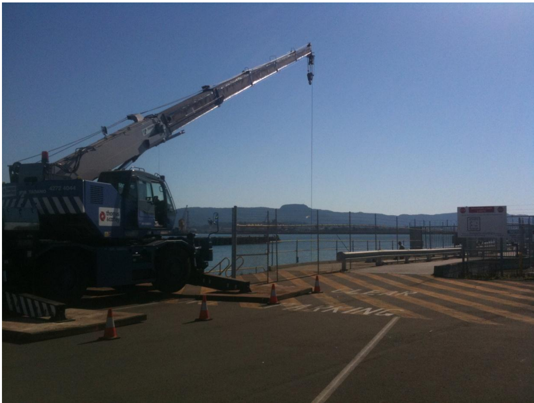
Figure 20: Sea crane provided by Thomas & Coffey
