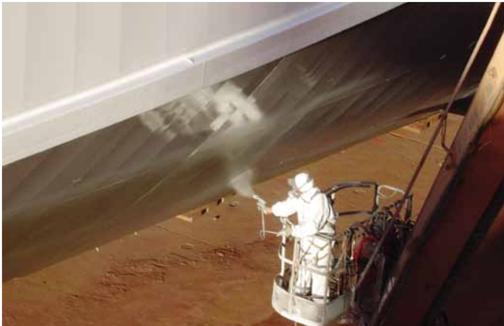
Antifouling paint application on a vessel in drydock
