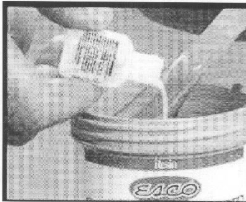
Figure 613-1-29A. Mixing of the SOCKETFAST Catalyst to Resin Mixture.
