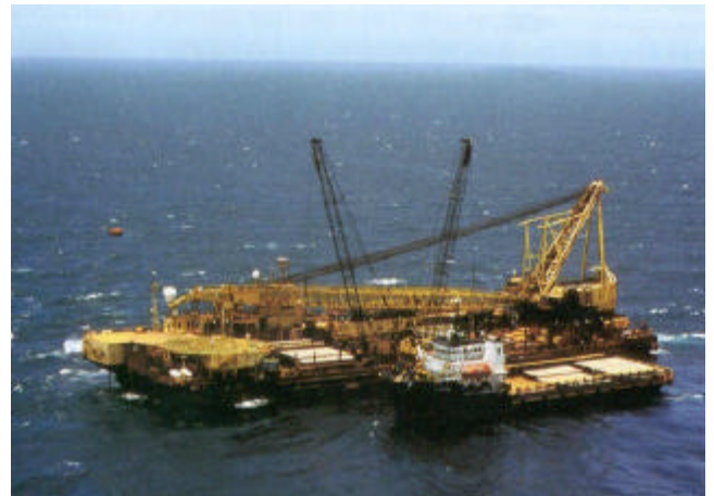
Fig.1. BGL1 with a supply boat at portside.
