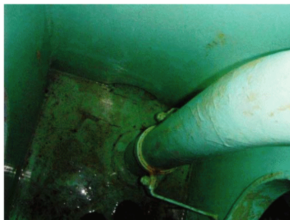
B. Waster (Doubler) Installed on Structure
