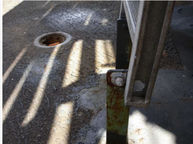
Aluminum Ladder and Steel Supports
