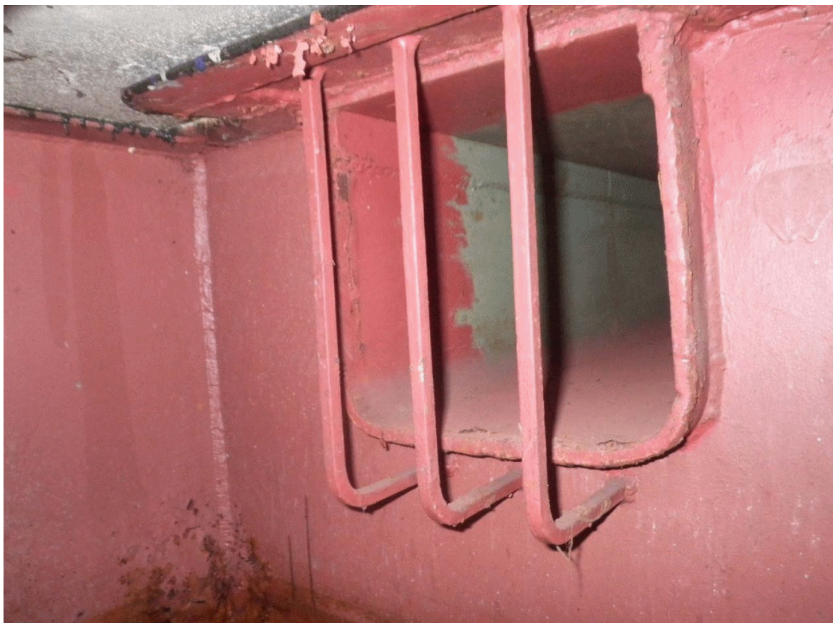
Figure 4-2 Opening to a Cross-Flooding Duct on CG-47 Class Ship
