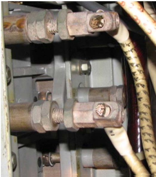
Figure 3-4. Two Possible Styles of Compression Type (DOSSERT) Cable Lug Connectors and Make-up to Circuit Breaker/Fuse Clip Current Stud
