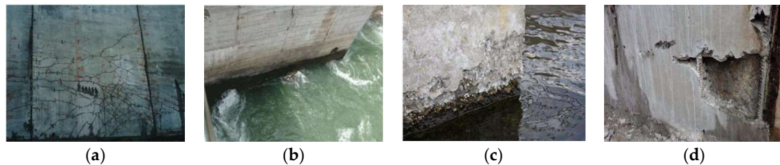
Figure 1. The common defects observed in the dam bodies of hydropower stations include (a) cracks, (b) water leakage, (c) surface erosion, and (d) tendon leakage.
