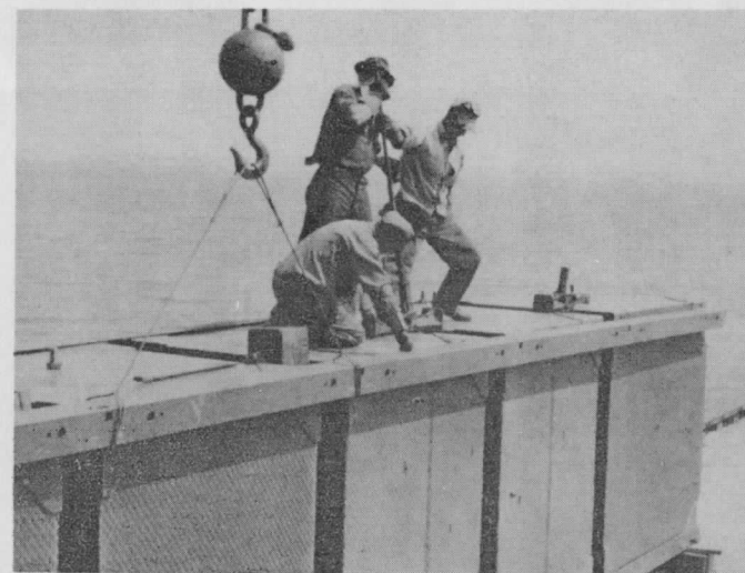
Fig. I-4 Pontoons being jacked at the top to allow the top assembly angles to fall into place.
