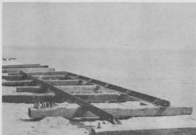
Fig. I-1 Assembly angles properly placed for pontoons.
