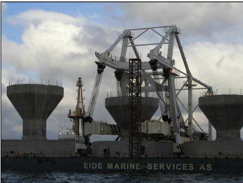
(b) Gravity Bases being lowered from barge
