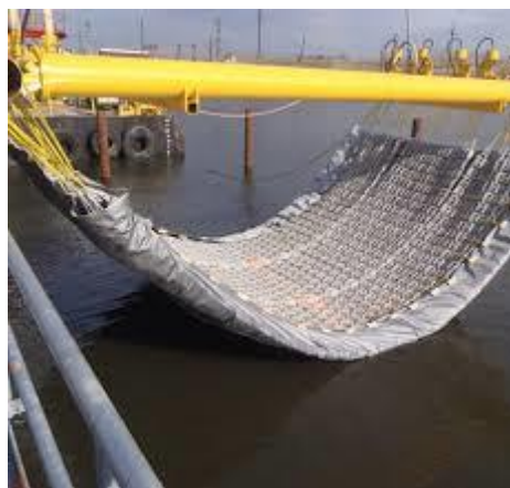
Figure 12. Scour protection concrete mattress
