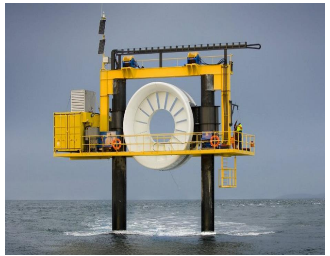
Fig. 2 Rim-driven generator, DCNS-OpenHydro. Image source [8]
