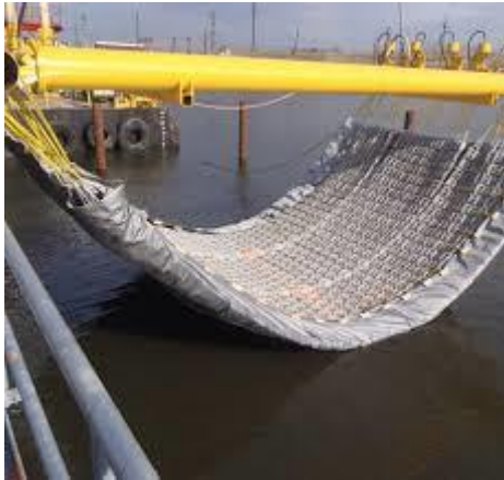
Figure 10. Scour protection concrete mattress
