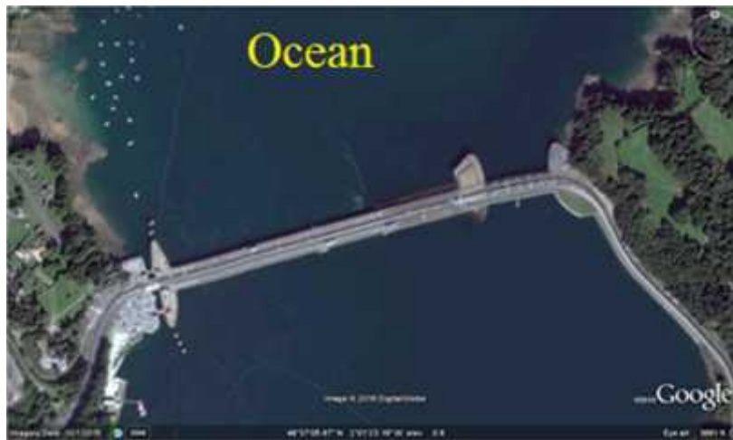
Figure 1. Top view of La Rance tidal power plant barrage (750m in length)
