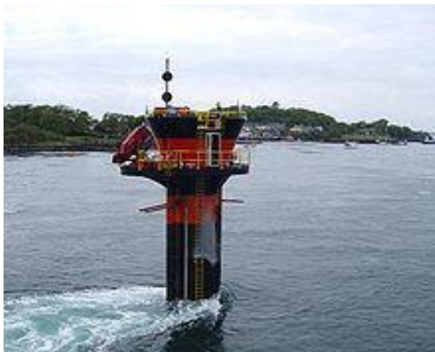
Fig. 1. The world's first commercial-scale and grid-connected tidal stream generator.
