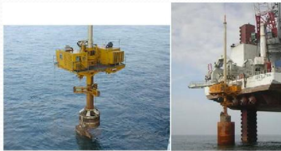
Fly-Drill 5500 Barrow Wind Farm. Source: Bauer Renewables
