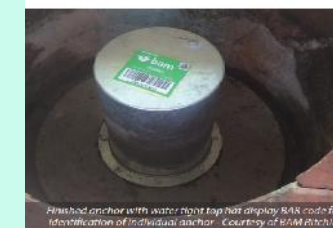
Source: BAM-Ritchies. Loch Arklet Dam Anchor Heads
