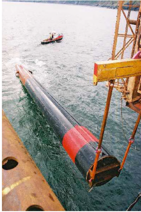
Figure 13: Semi-buoyant lift of pile into the casing.
