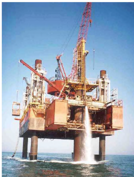
Figure 12: Seacore's Deep Diver jackup barge drilling the socket for the Seaflow foundation.
