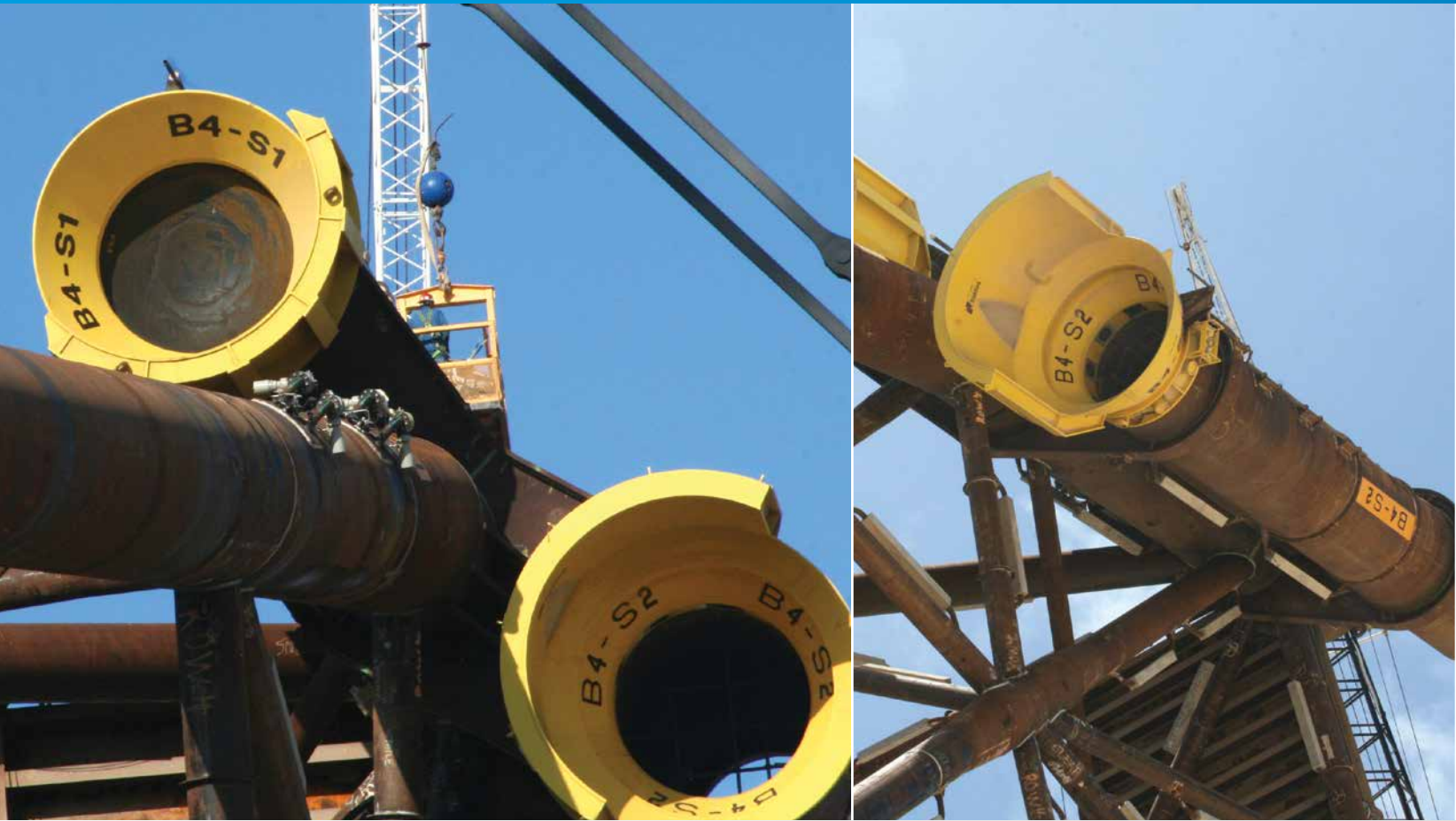
Buoyant Skirt Pile Sleeves with Integral Skirt Pile Gripper and Latch-Rings for Latch-Lok Leveling
