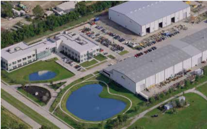
Houston Hobby Facility
