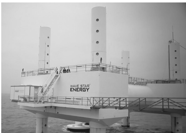
Fig. 8. Wave Power Plant Wave Star , Hanstholm, Denmark [18]
