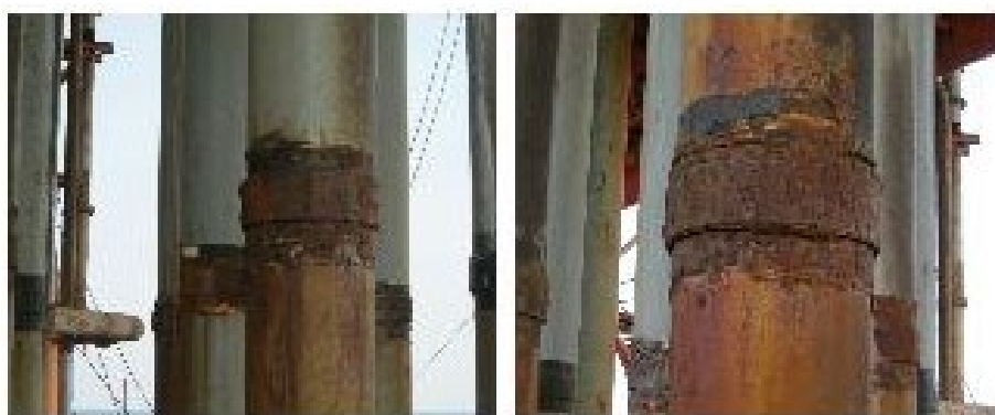
Figure 1. Corrosion conditions at casing joint locations.
