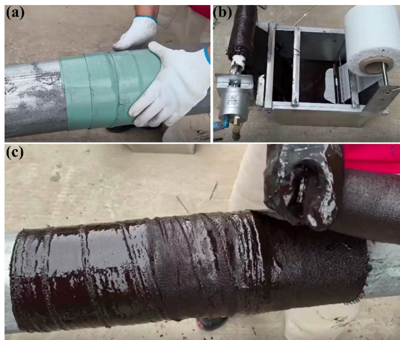
Figure 9. Application experiment on offshore oil and gas well conductor. (a) Internal protection material, (b) Coated high-strength fiber tape, and (c) Wrapped nano-polymer epoxy material.
