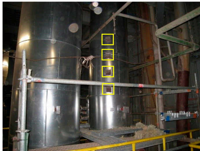
Figure 5. Holes in the insulation for measuring pipeline vibrations.
