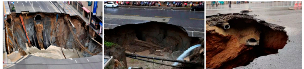
Figure 1. Collapses caused by pipeline leakage.
