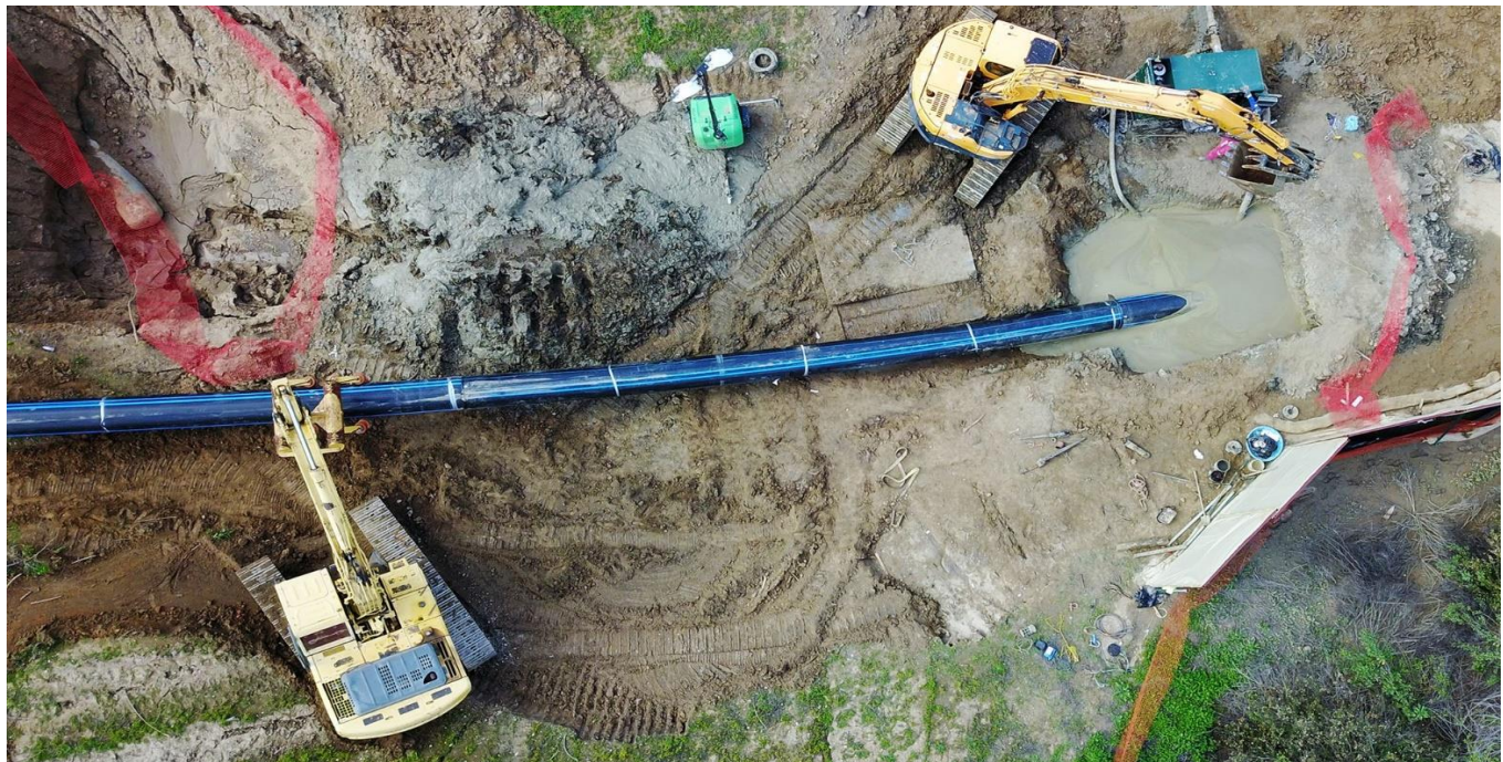
Fig 7. Aerial view of HDD Process [21]
