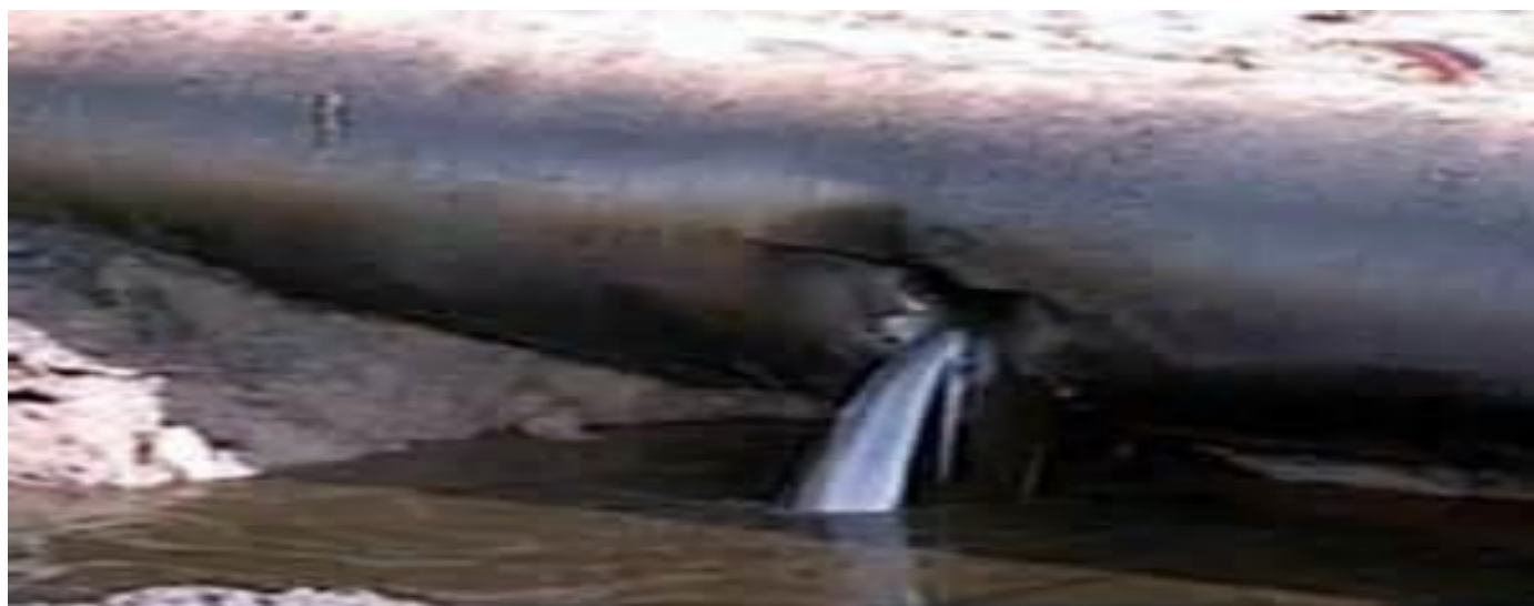
Fig 3. A crude oil line punctured by vandals [10]
