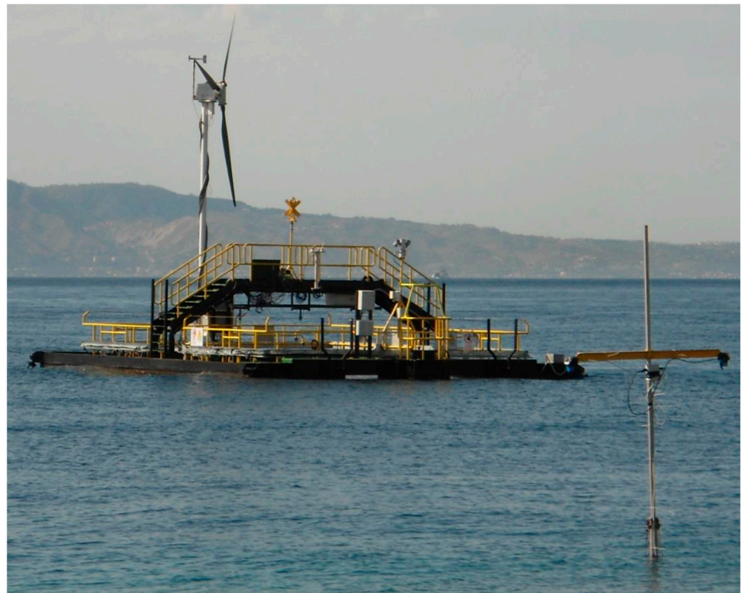
Figure 1. Photo of BGF platform installed at NOEL.
