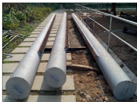
Fig. 2. Pile leg with gear rack
