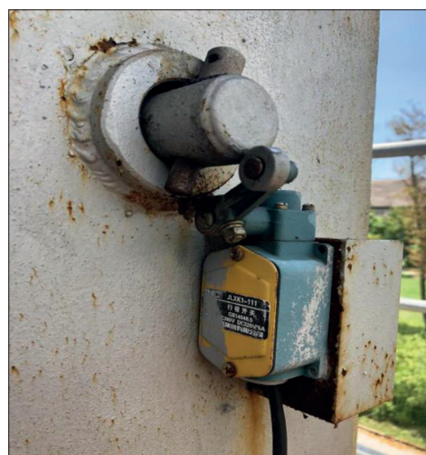
Fig. 4. Locking device
