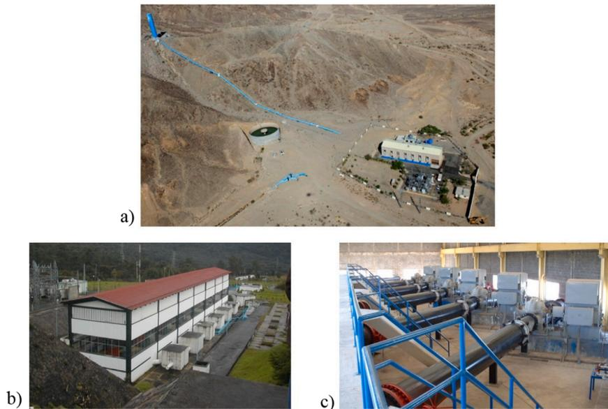
Fig. 1. Pumping station: a) Aerial view of a pumping station, pipeline, and standpipe; b) Thrust blocks in a manifold; and c) Pumps and their bases.
