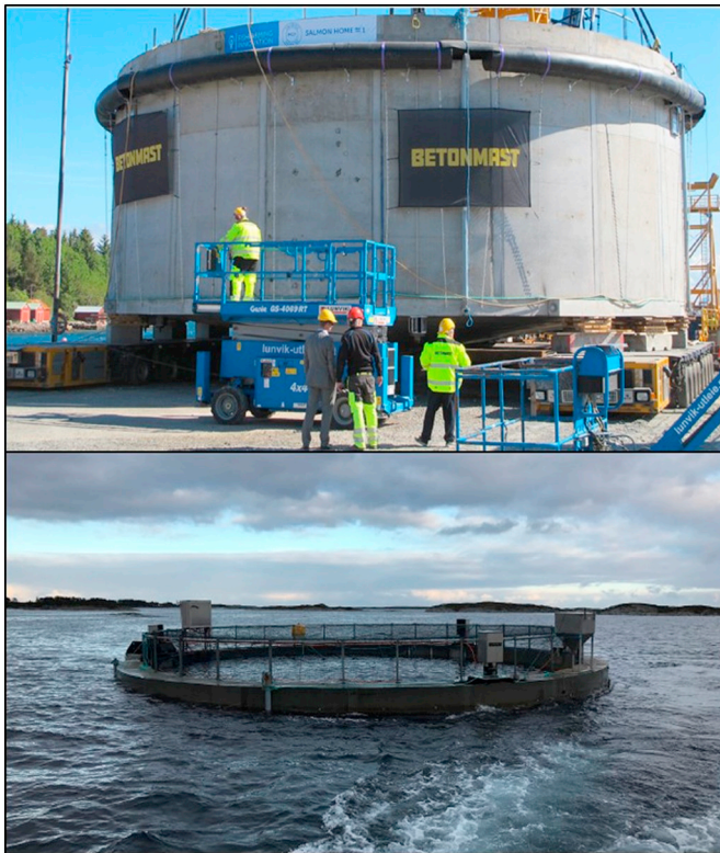
Fig. 26. Concrete containment fish tank (Picture courtesy of Tor Ole Olsen).
