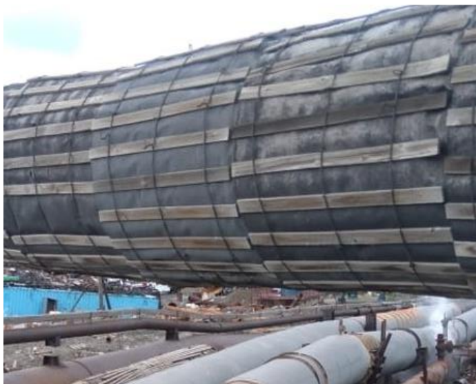
Fig. 1. The current state of aboveground pipelines
