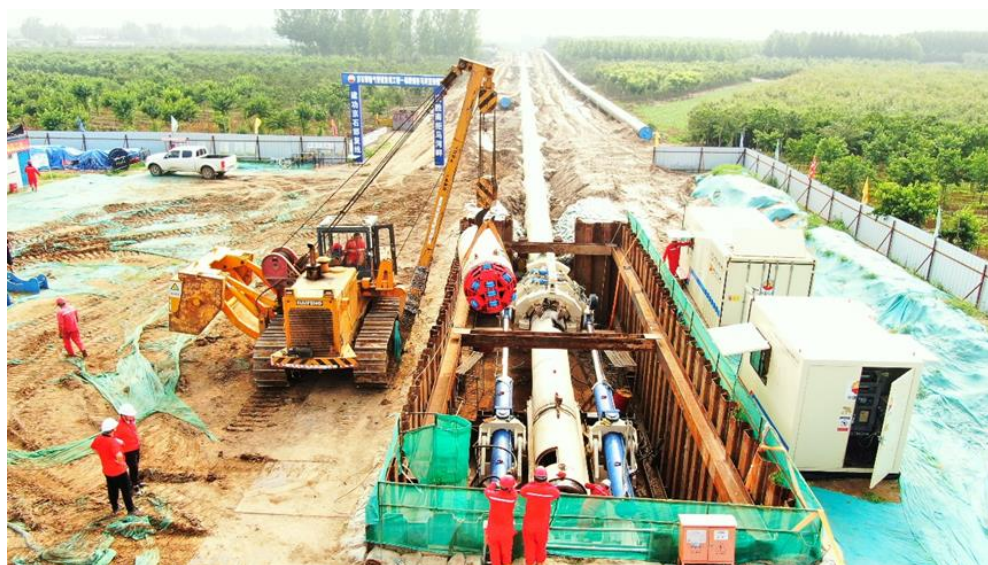
Figure 2. Figure of overall layout of construction site.
