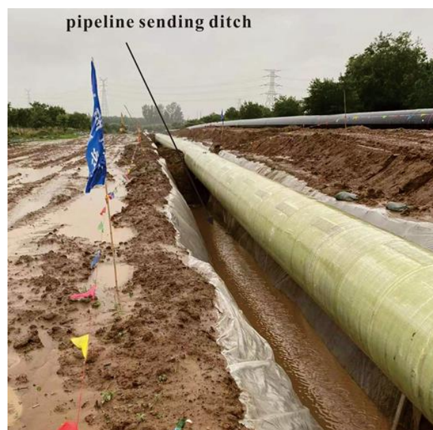
Figure 14. Pipeline sending ditch.
