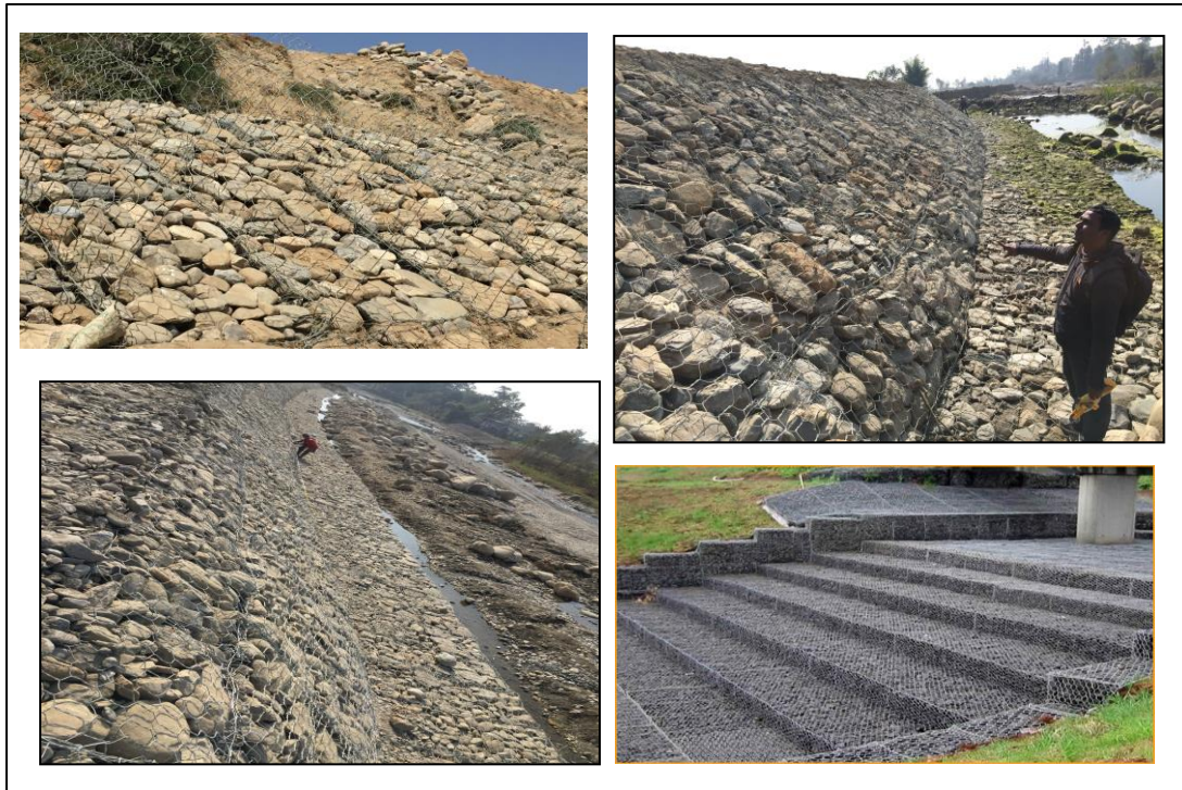
Figure 14. Completed installation of gabion mattress for the river bank protection.
