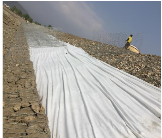
Figure 2. Geotextile installing below gabion mattress at slope.
