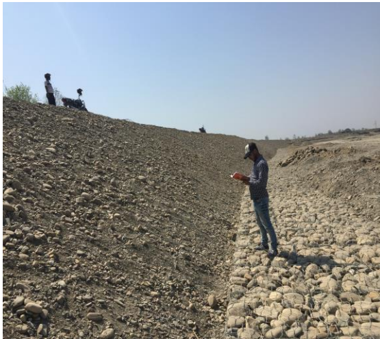
Figure 1. Observation of slope before installing gabion mattress.
