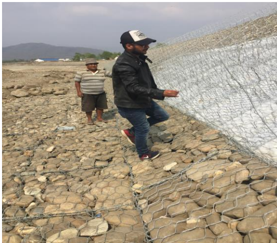
Figure 3. Inspection of work at slope area.
