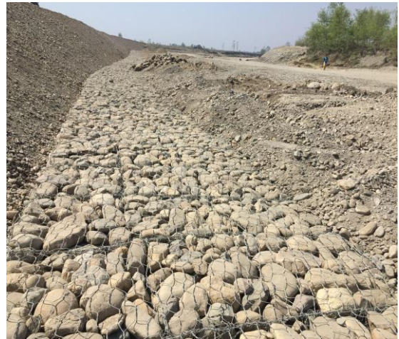
Figure 4. Installed Launching apron.
