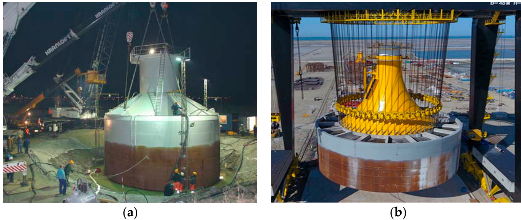
Figure 1. The prototypes of wide-shallow bucket foundation: (a) Frederikshavn, Denmark [17]; (b) Xiangshui, China.
