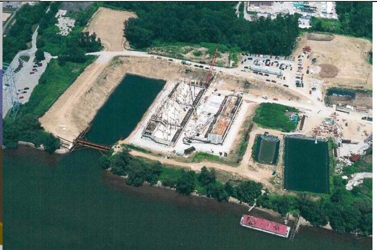
Clockwise from upper left: Launch and 10-mile tow of first dam segment from casting basin to upstream outfitting and installation site at Braddock, PA; first dam segment being positioned at site prior to ballasting down onto pre-installed foundation and concrete filling; schematic of first dam segment being ballasted down for mating to pre-installed river bed foundation; cast yard and two-level launch basin.
