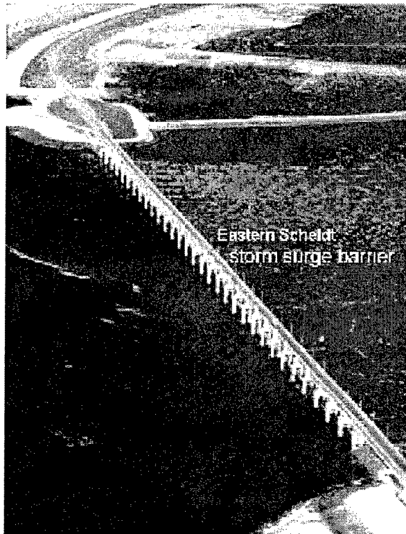
a. Storm surge barrier
