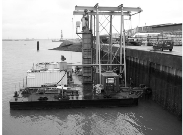
Figure 4, Limpet and gantry on a barge
