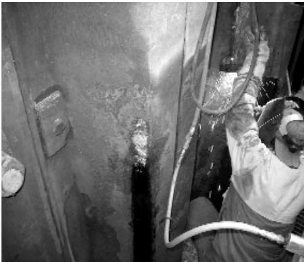
Figure 8. Sealing wet holes
