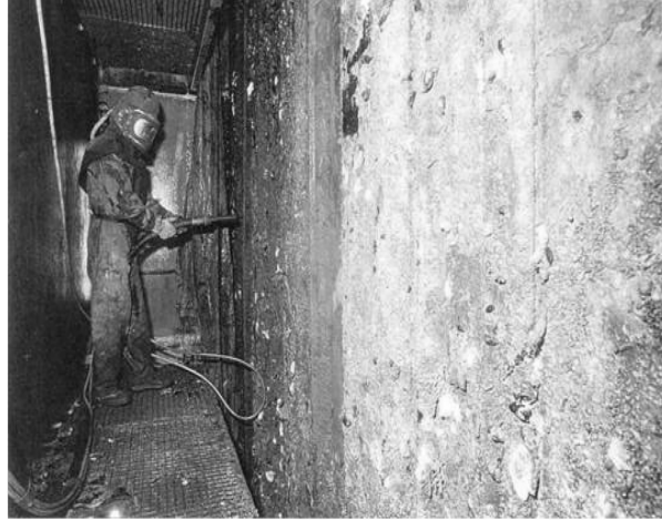
Figure 7. Abrasive blast cleaning inside a limpet
