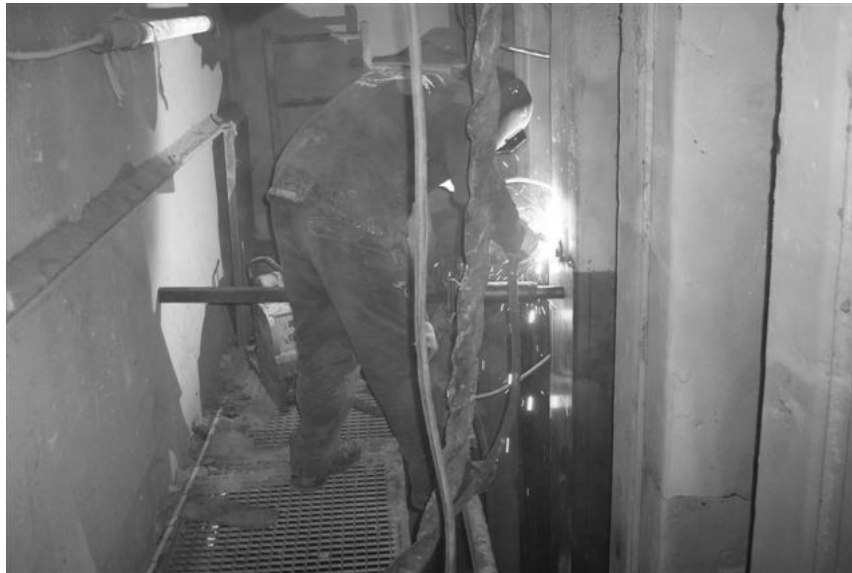
Figure 1. Worker repairing steel sheet piling in a limpet cofferdam
