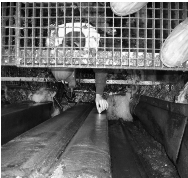
Figure 5. Structural inspection for steel thickness and holes
