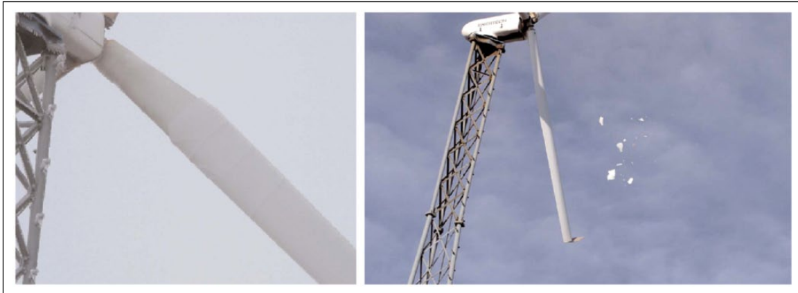
Figure 11. Ice accumulation and falling off on a wind turbine at Wachusett Wind Power (WindAction, 2012).
