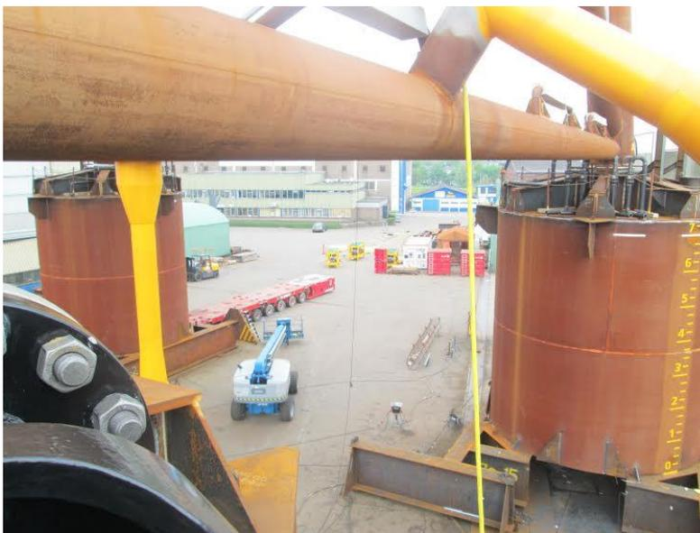
The buckets are 7.0 m in diameter, and have a total length of 7.4 m. The embedded depth is less than the shell length, this is to account for loosening of the soil inside the bucket. After installation a grout mixture was inserted to fill the space between soil and top plate inside the bucket. The structure was installed in water with a depth of about 20 m. At the location
