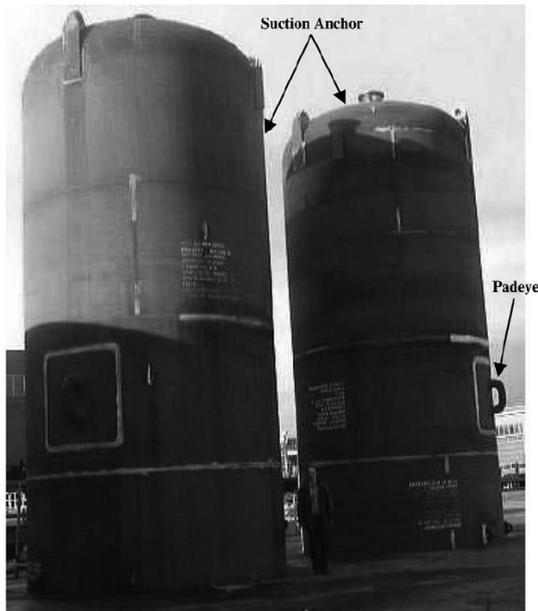
Typical suction anchors possess very high ratios of diameter to wall thickness ( $d/t$ ) ranging from 100 to 250. In the skirt wall, internal stiffeners are included to prevent buckling of the structure during the installation and due to mooring loads during operation (Randolph et al, 2005).
