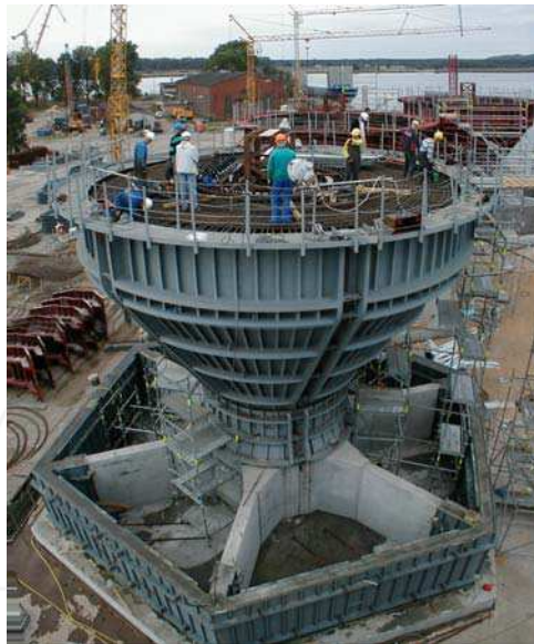
Fig. 7. Gravity Base Foundation being constructed for Nysted Offshore Wind Farm at Rødsand, Denmark. (Courtesy of Bob Bittner, Ben C. Gerwick, Inc.)
