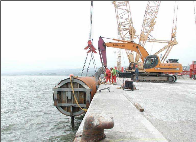
(a) Monopile being floated out to site.
