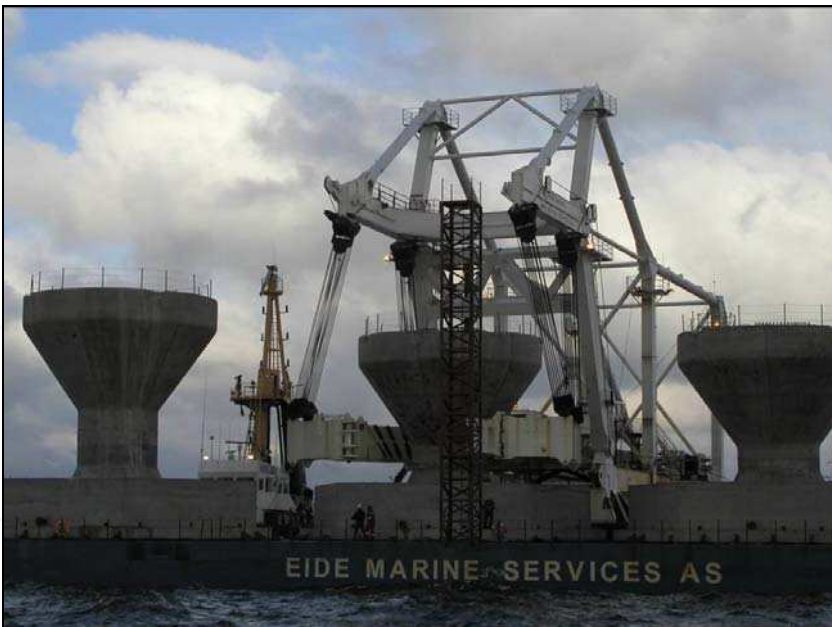
(b) Gravity Bases being lowered from barge
