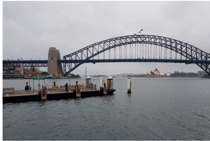
Figure 1. A ferry commuter floating pontoon located at McMahon's Point in Sydney Harbour, Australia.
