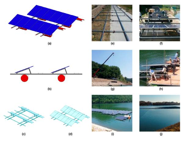
**Figure 14.** Floating photovoltaic system: (**a**) unit module, (**b**) side view, (**c**) frame, (**d**) photovoltaic, (**e**) basic frame assembly, (**f**) photovoltaic module installation, (**g**) lifting, (**h**) launching, (**i**) assembly on water surface, and (**j**) completion.
