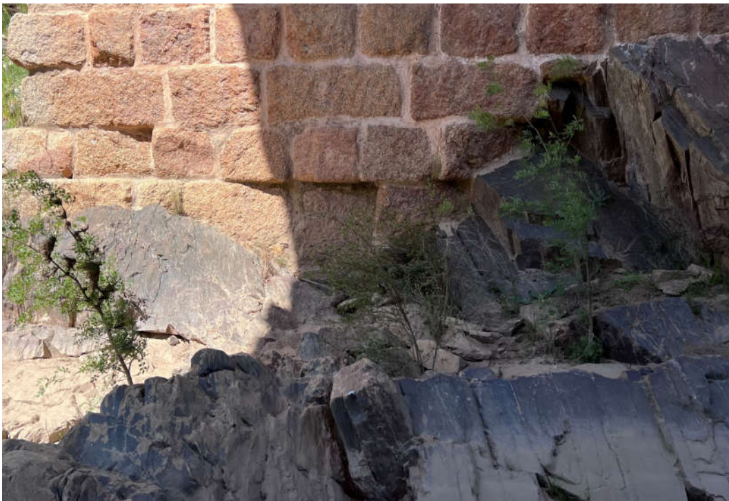
Figure 3. Close-up of the abutment on the Portuguese side, showing the arrangement of its first rows on the rocky material (photo by the author).
