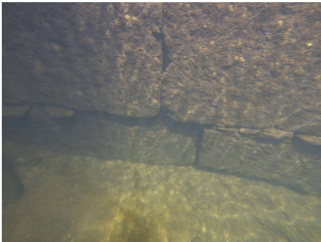
Figure 13. Condition of another fragment of the lower part of one of the inspected piles, in an image captured by the underwater drone (photo by the author).
