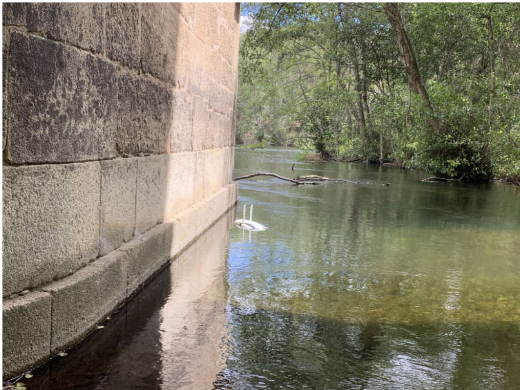
Figure 9. Underwater drone approaching one of the central piers of the San Lorenzo Bridge from downstream (photo by the author).
