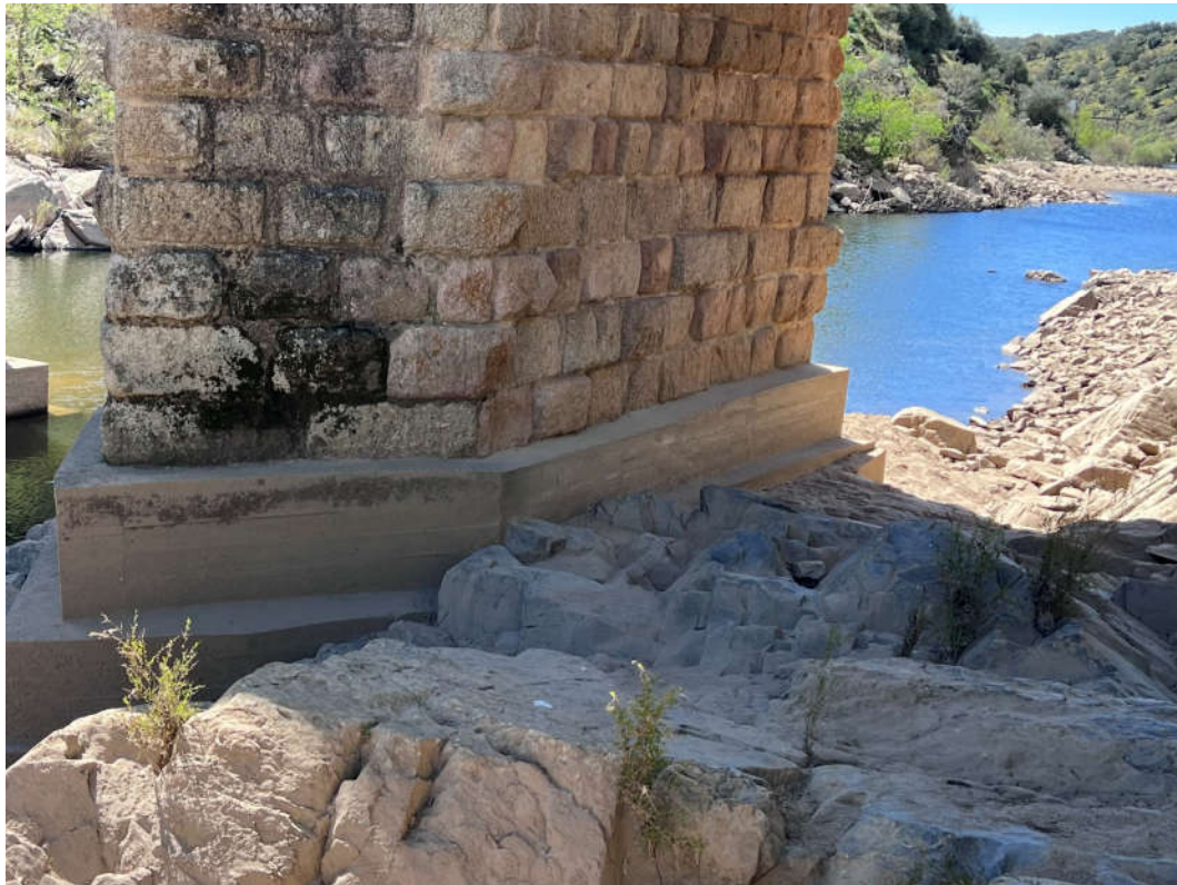
Figure 4. First pile, starting from the Portuguese side, where the casing and supporting rock can be seen (photo by the author).
