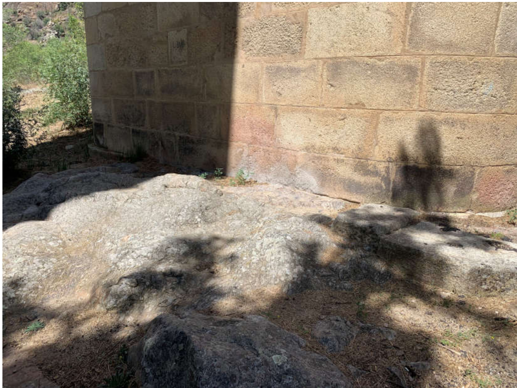
Figure 10. View of the first pier of the bridge, counting from the northern abutment (Zamora side), showing its support (photo by the author).
