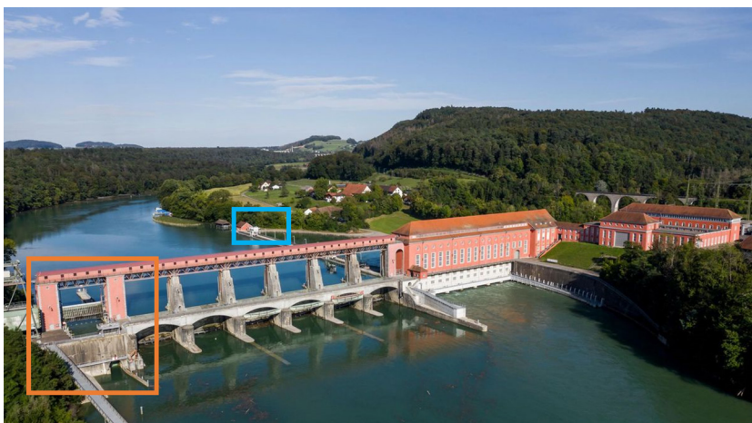
Fig. 3 The Hydropower plant in Eglisau: The water lock (orange) and the water filter (blue) in the inlet basin.
