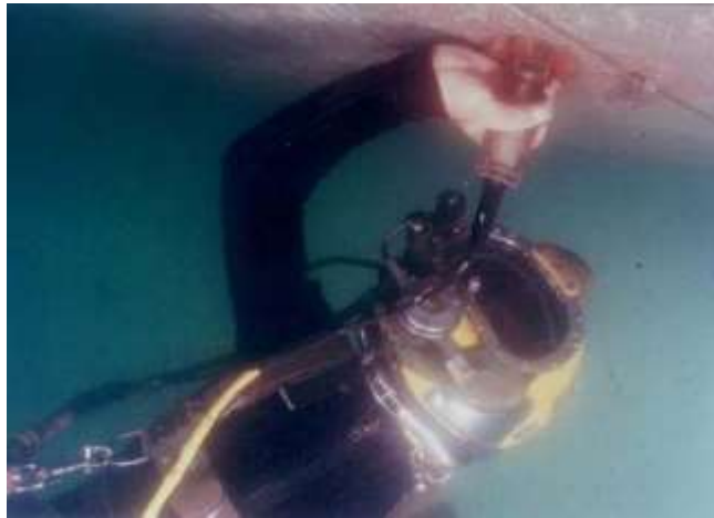
Figure 7. UT - Ultrasonic Testing under water (Hedayati, 2010)
