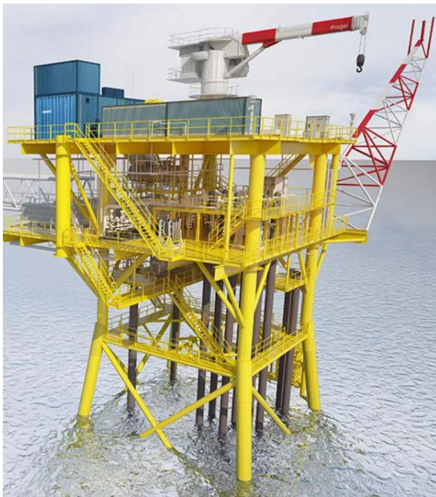
Figure 2 Example of offshore Jacket platform
