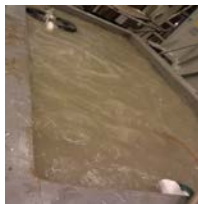
Figure 4: The photo showing the tank and muddy water content
