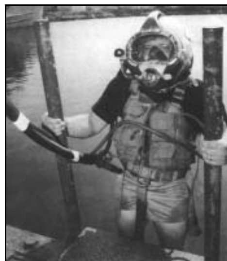
Figure 8-1. MK 21 MOD 1 SSDS.
