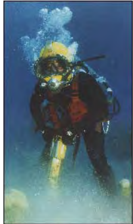
Figure 6-4. Underwater Construction Diving.
