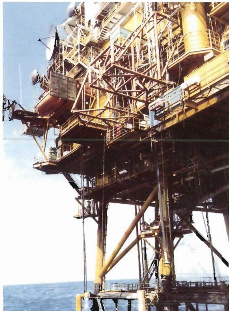
Plate 10(b) The north-west corner of the platform, showing the Chanter riser gantry. The gantry is the two structures, one ending in a triangular shape and the other in a rectangular one, projecting from the 68ft level. Also shown is the 20ft level and the navigation aid platform at the north-west corner of the 68ft level.
