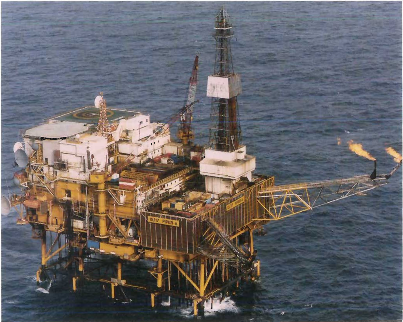
Plate 5 The Piper Alpha platform: west face and pipe deck.
