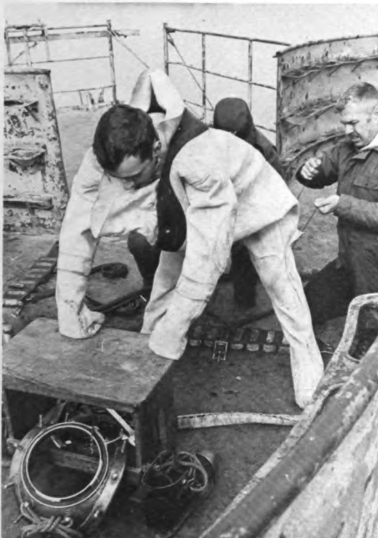
E While the diver supports himself on a bench, the tenders lace the suit.
