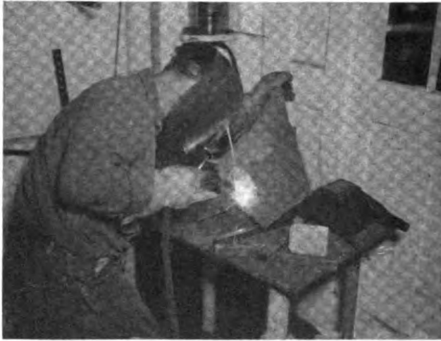
PLATE 5—FIGURE 1.—Training in above-water burning as a prelude to under-water cutting.
