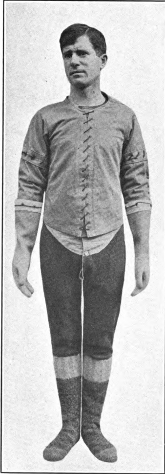
DIVER PARTLY DRESSED, SHOWING UNDERJACKET WITH RUBBER GLOVES ATTACHED.
