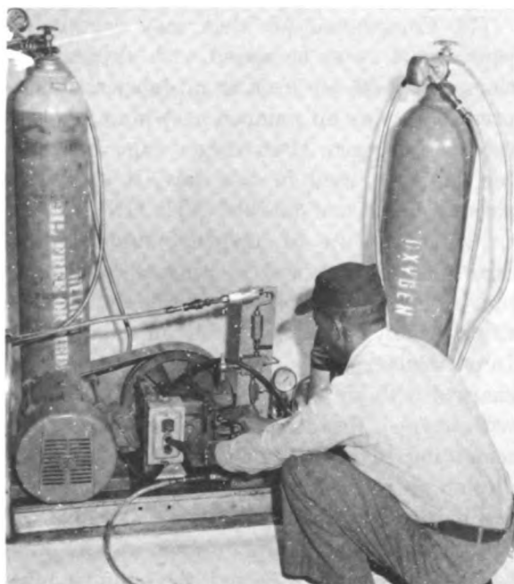
FIGURE B-1.—Oxygen-transfer pump.
